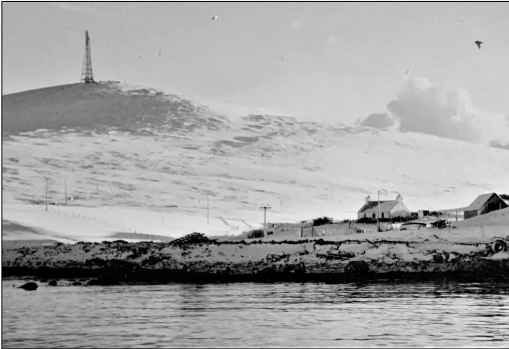
The Ward of Bressay transmitter in the big snow at Christmas 1995.
